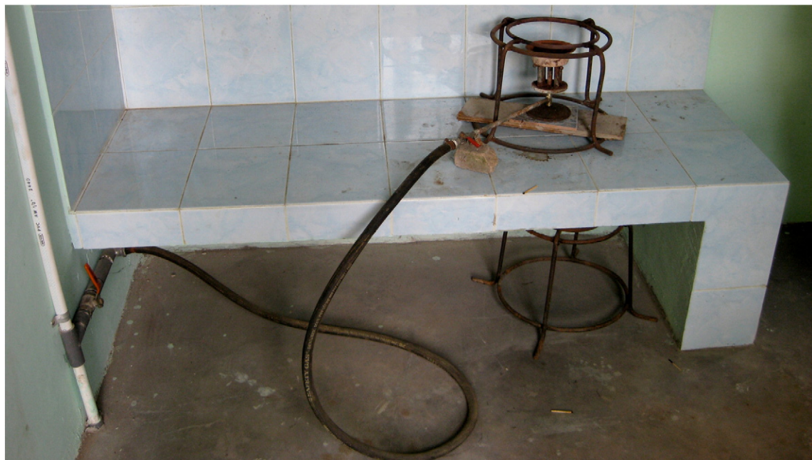
Fig. 3. Biogas stove, Java, Indonesia (picture: Elisa Roma, University of KwaZulu-Natal, South Africa).
