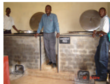
Institutional rocket stove at Nyamnina Pr. School in Sauri Millenium Village – Yala
