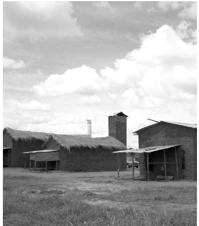
Figure 4 Rocket Barns cure tobacco more efficiently, Malawi (Photo: GTZ)
