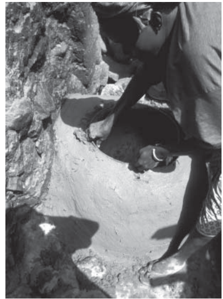
Figure 7 Rotating and lifting it at the same time the embedded cooking vessel is carefully removed. (photo: Peeyush Sekhsaria)
