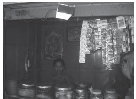
Figure 3 Woman entrepreneur - SELCO installation (photo: ITPI personnel)
