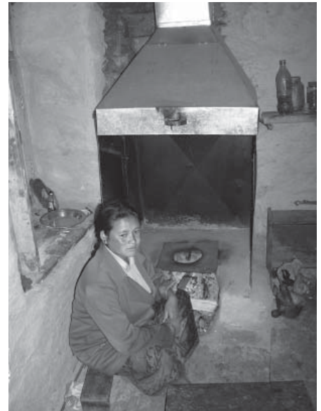
Figure 2 Woman sitting beside improved stove with smoke hood: house with insulated walls (photo: Practical Action UK)
