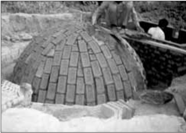
Figure 2 Biogas plant installation (photo: Rakesh Prasad)
