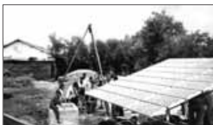
Figure 4 Solar water pump installation in Harpalpur village (photo: Rakesh Prasad)
