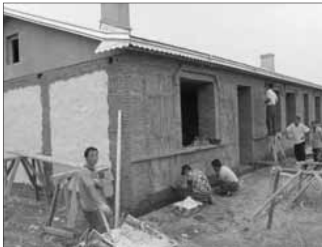
Figure 2 Straw bale walls
