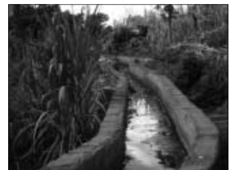
Figure 1 Micro-hydro scheme at Chuka, Mbuiru Village. Canal taking water from the river to the penstock and then the power house (photo: ITDG East Africa)
