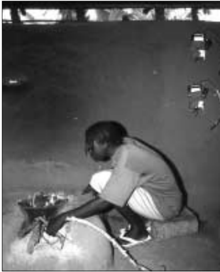
Figure 3 Eaves spaces and Upesi stove installed in West Kenya (photo: Nigel Bruce)
