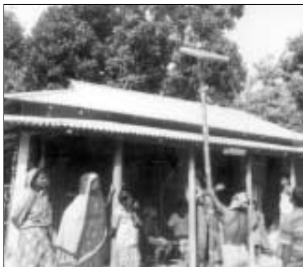
Figure 4 Installing a solar home system
