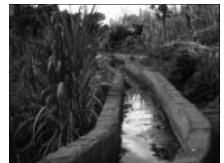
Figure 1 Micro-hydro scheme at Chuka, Mbuiru Village. Canal taking water from the river to the penstock and then the power house (photo: ITDG East Africa)
