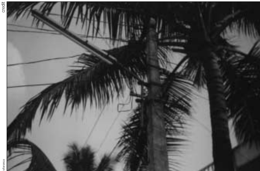
Figure 2: Illegal 'hook up' to electric supply
